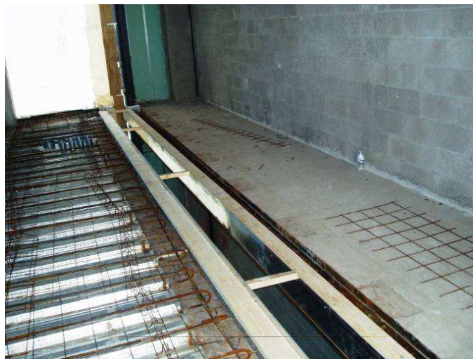
Figure 5 - Expansion Joint Section Photo Courtesy Jim Boje, PE (Wendel)
